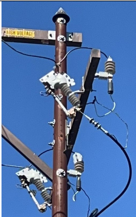
IA1img1: Missing avian protection on lightning arrester
