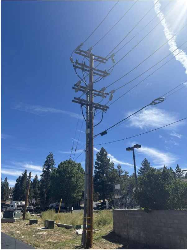
IA1Img1: View of new pole with no fire-resistant wrapping
