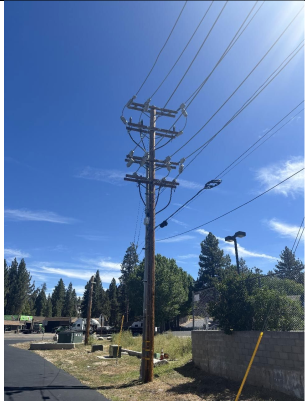
IA1Img2: View of new pole with no fire-resistant wrapping
