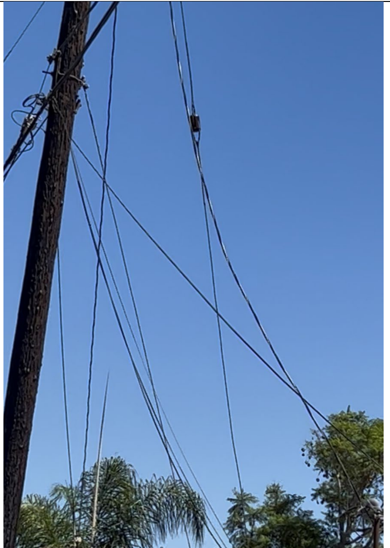
IA1Img4: View showing loose down guy
