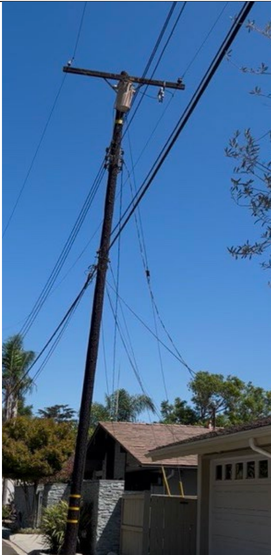
IA1Img3: View showing loose down guy
