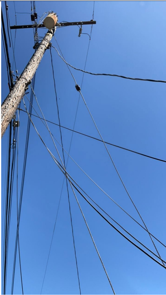
IA1Img1: View showing both down guy wires are loose
