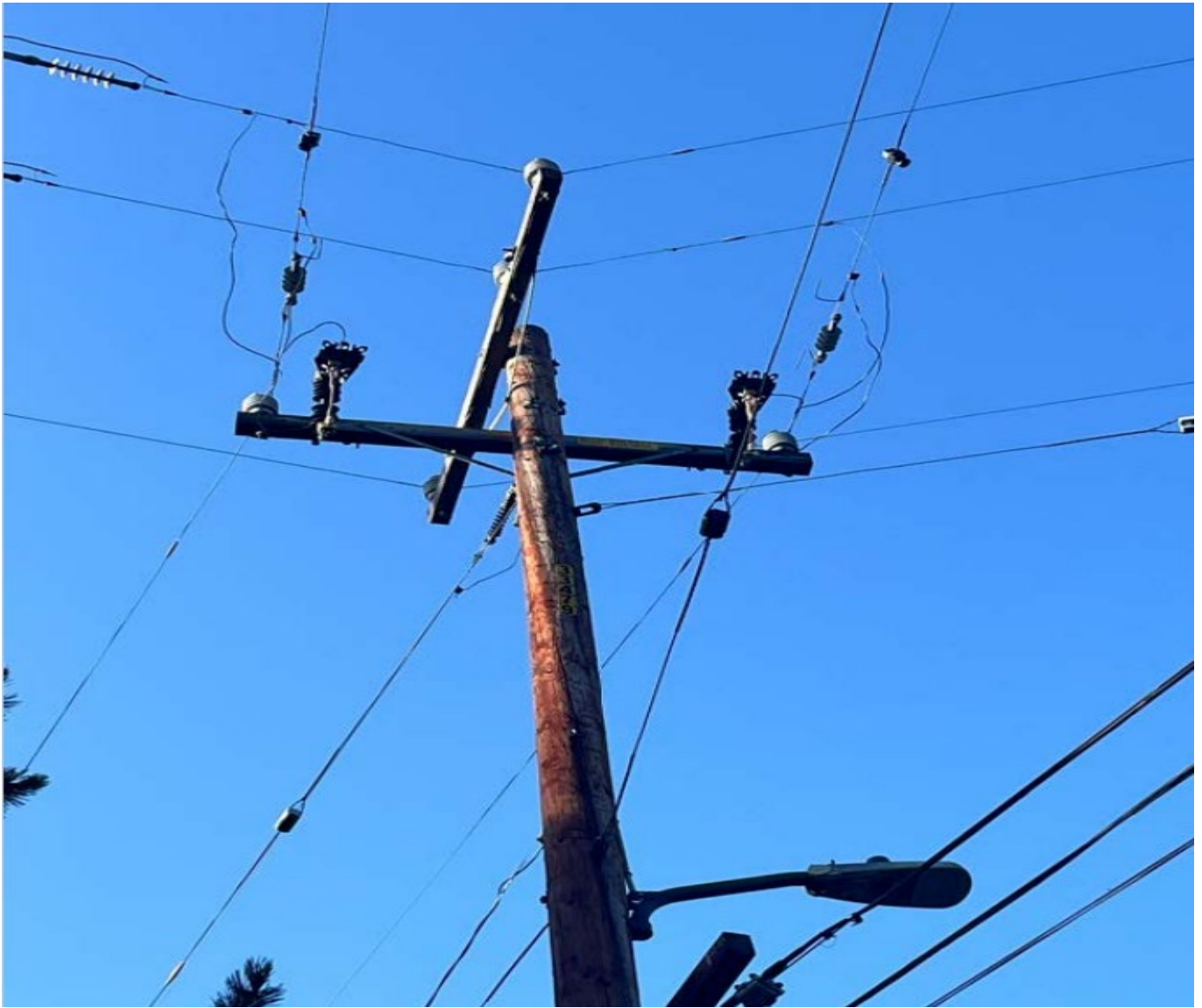
Image 2: Zoomed in view of pole ID 33479 with completed replacement Non-Exempt Expulsion Fuse with Solid Blades.
