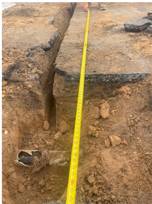
Photo 2: Photo taken and provided by Rancho's Curley of the distance between locate marks and the damaged facility. (Exh. 7.)
