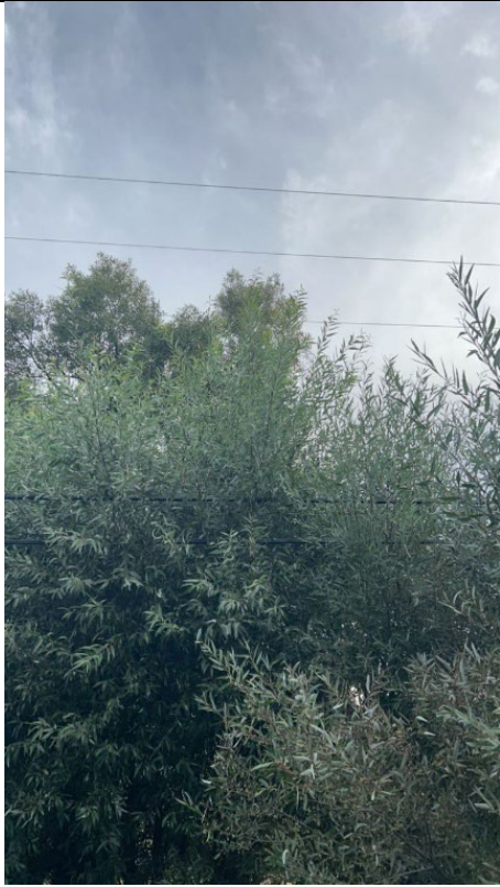
Photo 3: View of the tree branches located within 3 feet of the distribution line. The photo was taken facing northeast from the street.
