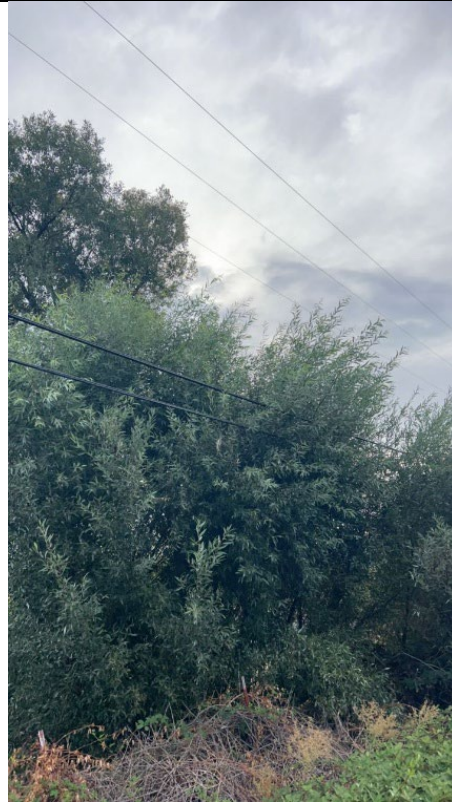
Photo 4: Secondary view of the tree branches located within 3 feet of the distribution line. The photo was taken facing east from the street.
