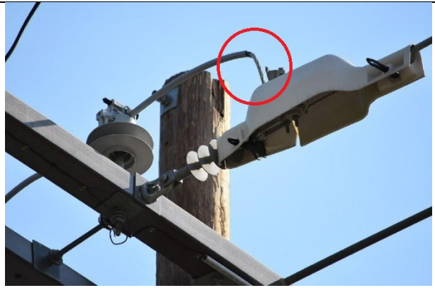
IA1Img4: Middle phase missing connector cover
