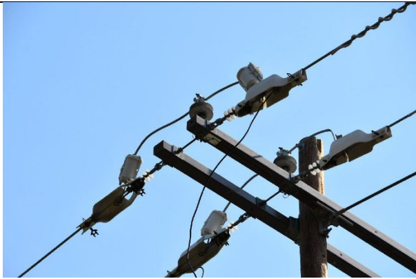
IA1Img3: Middle phase missing connector cover
