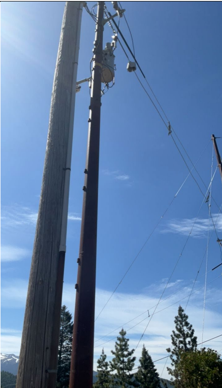
Item1IA1Img2: The newly replaced distribution pole and the old pole still in use as a riser support
