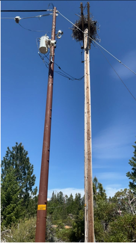
Item1GImg3: View of the newly replaced and the old distribution pole
