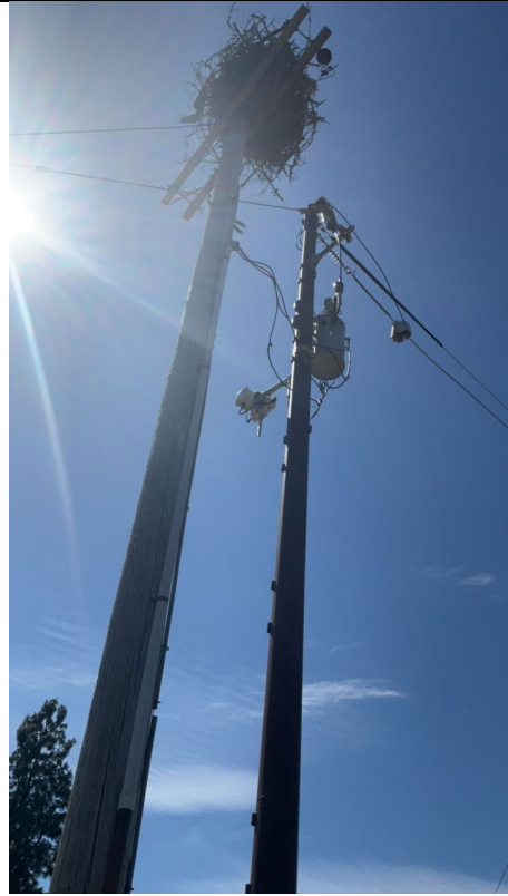
Item1IA1Img1: The newly replaced distribution pole and the old pole still in use as a riser support
