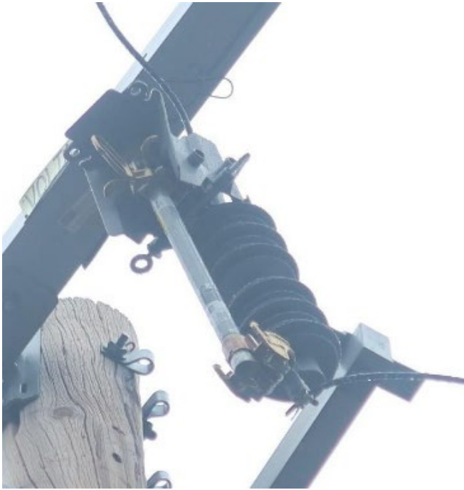
Item1IA1Img3: CalFire-exempt fuse is missing bottom-mounted red rain cap.
