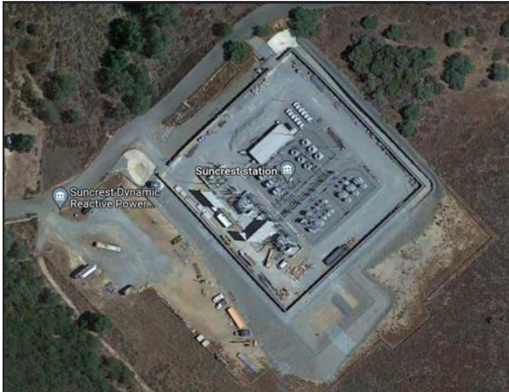
Figure HWT 4-2. Overhead Close-up of Suncrest SVC
