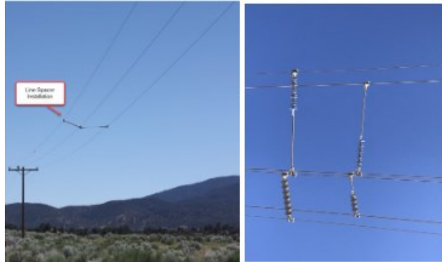
Figure SCE 8-05: A Line Spacer Installed on a Long Span to Mitigate Wire-to-Wire Contact (Left), Close Up Line Spacer View (Right)
