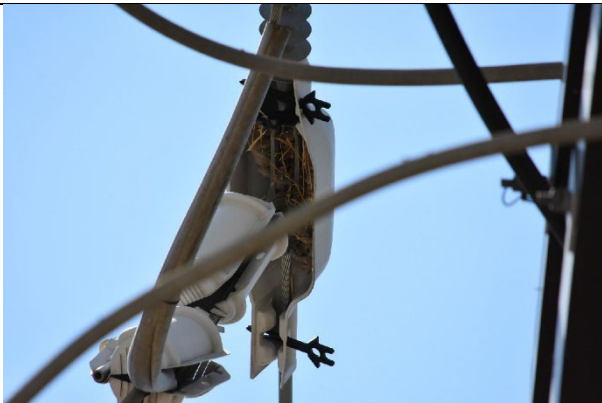
IA1img2: Bird nest observed in avian protection cover
