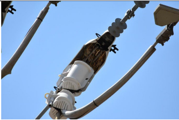
IA1Img3: Bird nest observed in avian protection cover
