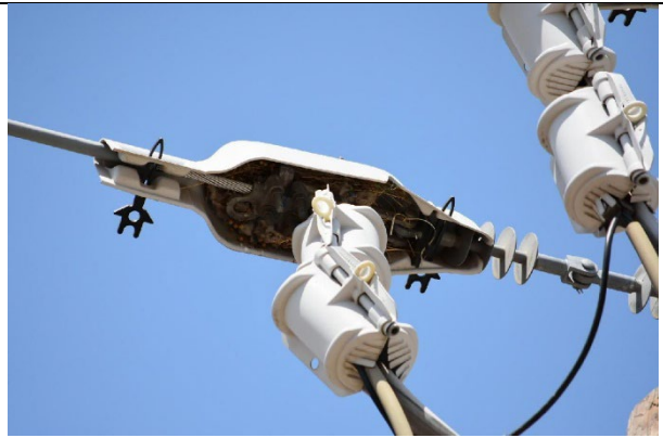
IA1Img4: Bird nest observed in avian protection cover
