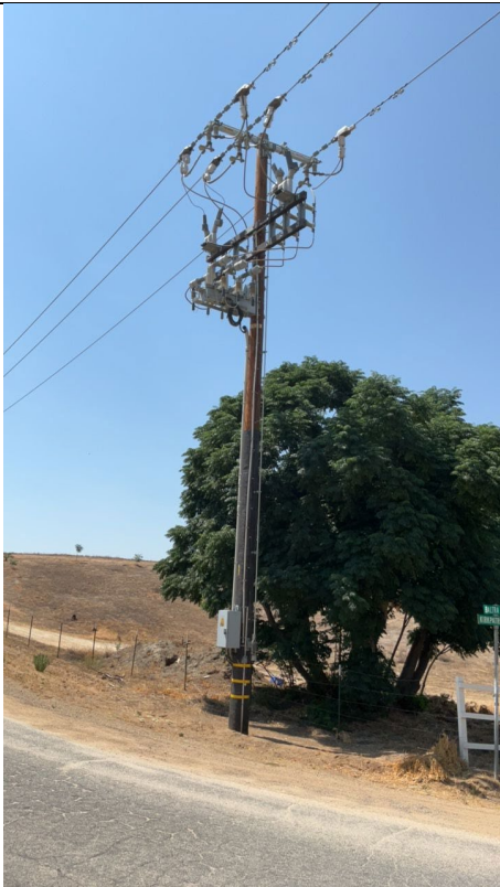
GIimg1: Overall Structure
