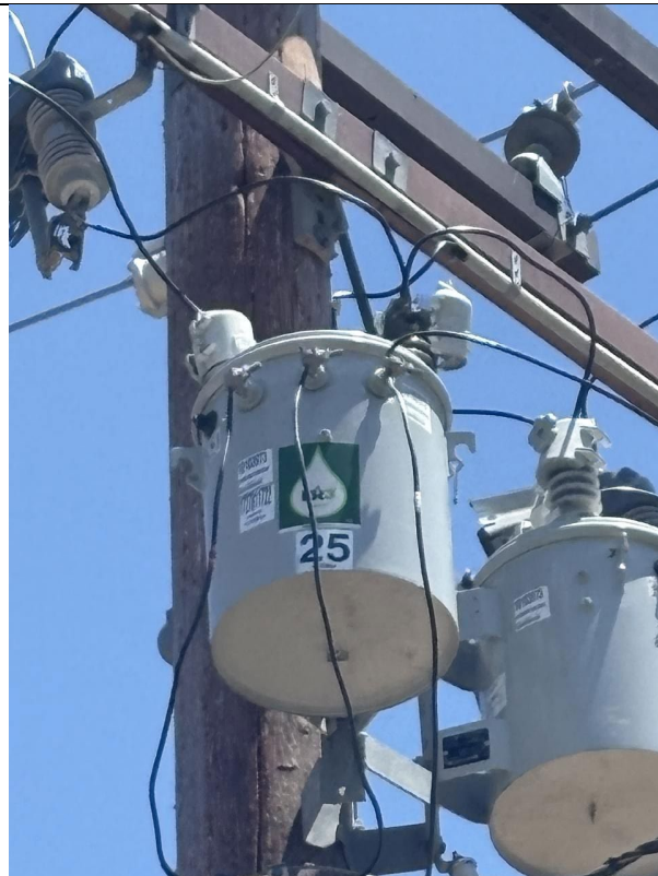
IA1Img3: Transformer bushings unhinged
