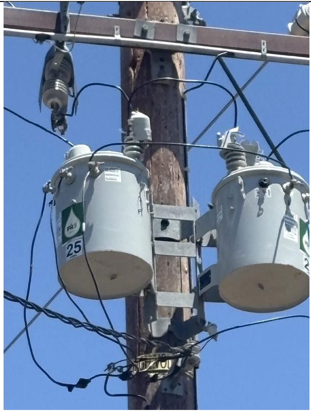
IA1Img2: Transformer bushings unhinged
