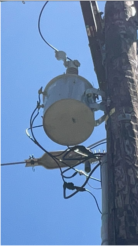
IA1Img1: View showing opened transformer bushing cover
