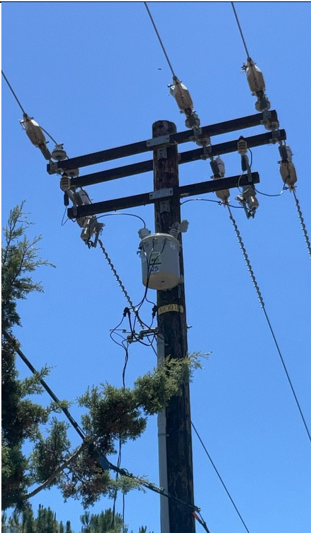
IA1Img3: View showing opened transformer bushing cover
