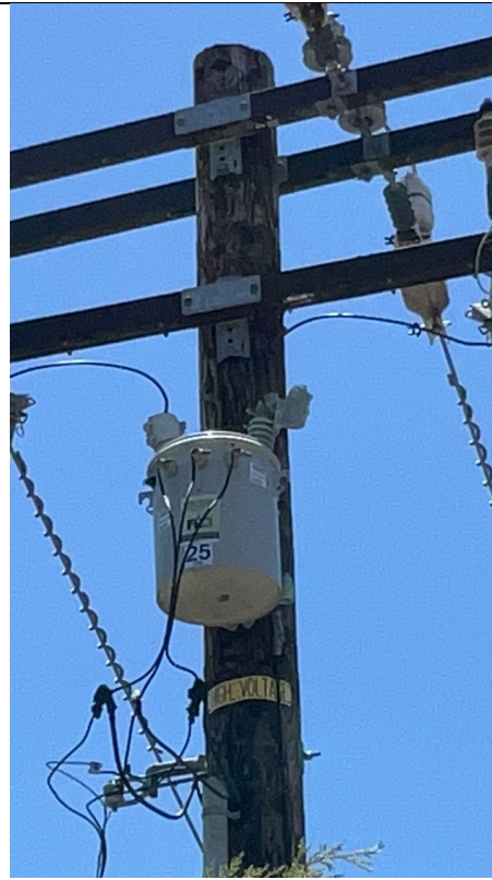
IA1Img2: View showing opened transformer bushing cover
