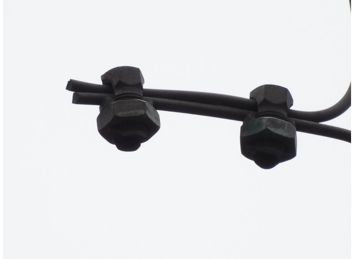
Item1IA1Img2: Closer view of the non-exempt split bolt connectors on the pole.
