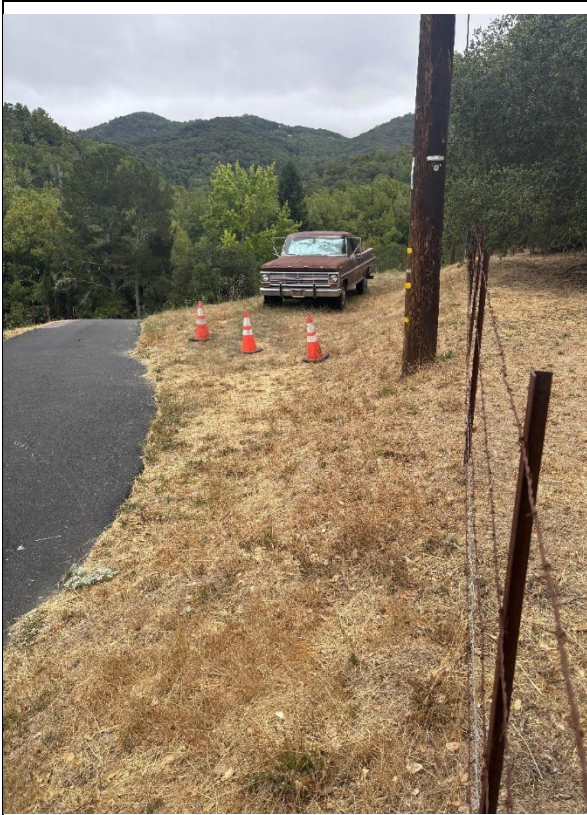
Item1IA1Img3: Dry flammable vegetation within 10-foot radial distance of the pole.
