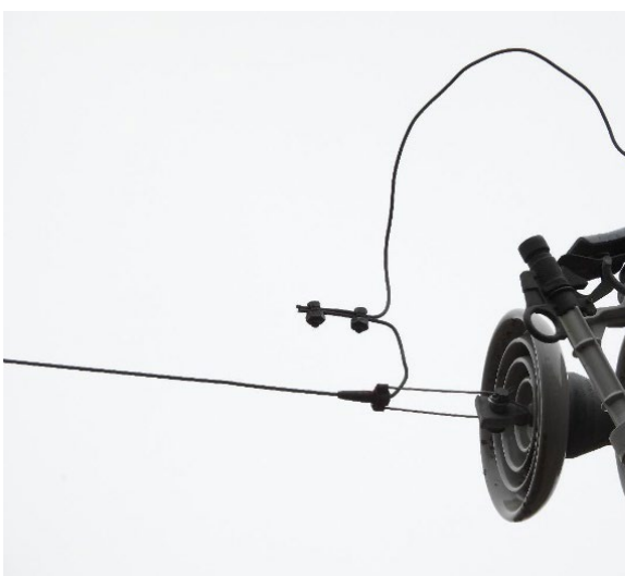
Item1IA1Img1: Non-exempt split bolt connectors on the pole.
