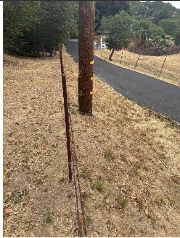
Item1IA1Img4: Dry flammable vegetation within 10-foot radial distance of the pole.
