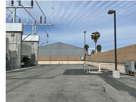
Pittsburg Station- Fire lane and 12ft perimeter wall
