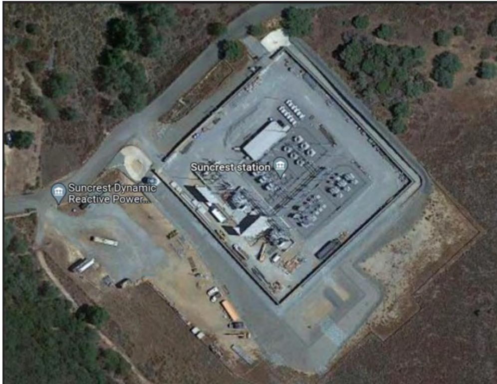
Figure HWT 4-2. Overhead Close-up of Suncrest SVC
