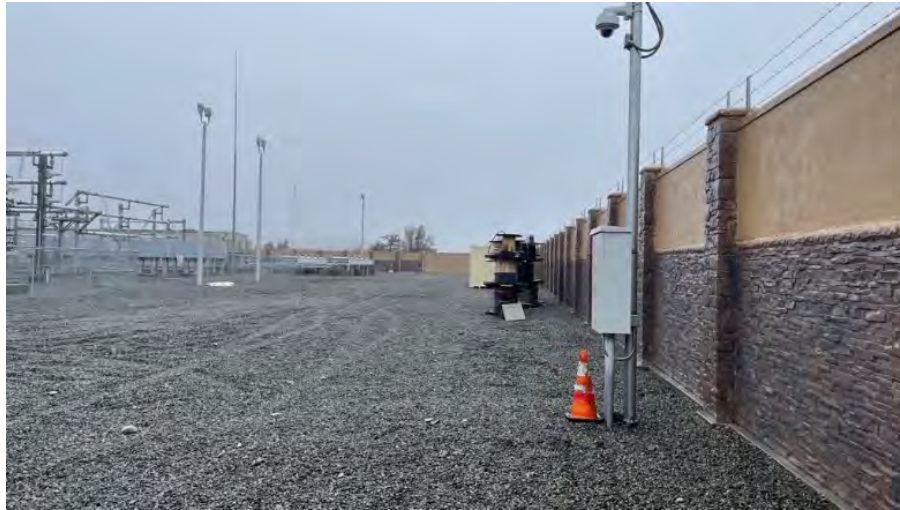
Figure HWT 10-1. Example of Site Camera
