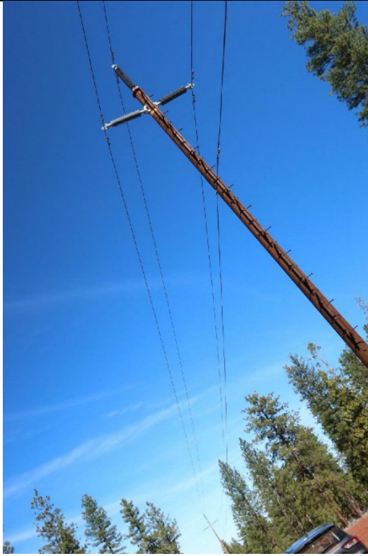
Item1IA1Img1: One of the spans with no existing splice
