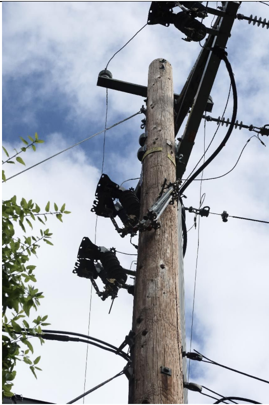
Item1IA1Img1: Exempt fuses hanging on pole and solid blade disconnects on cutouts.
