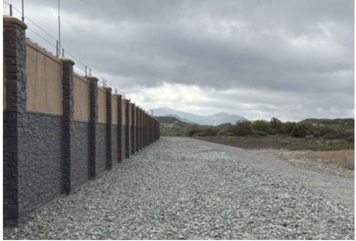
Firebreak Outside Exterior Walls
