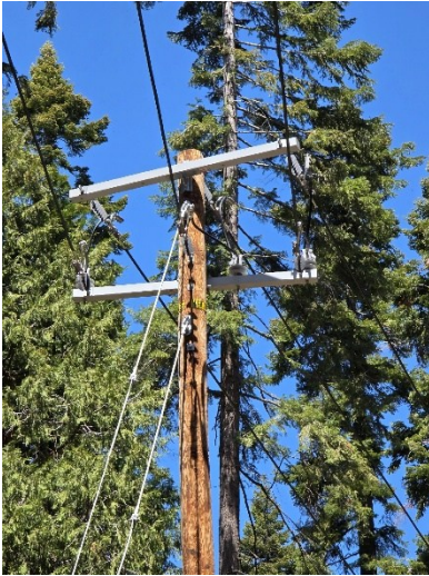
Figure 3: Example of Covered Conductor Installation (Foot Patrol) Field Images
