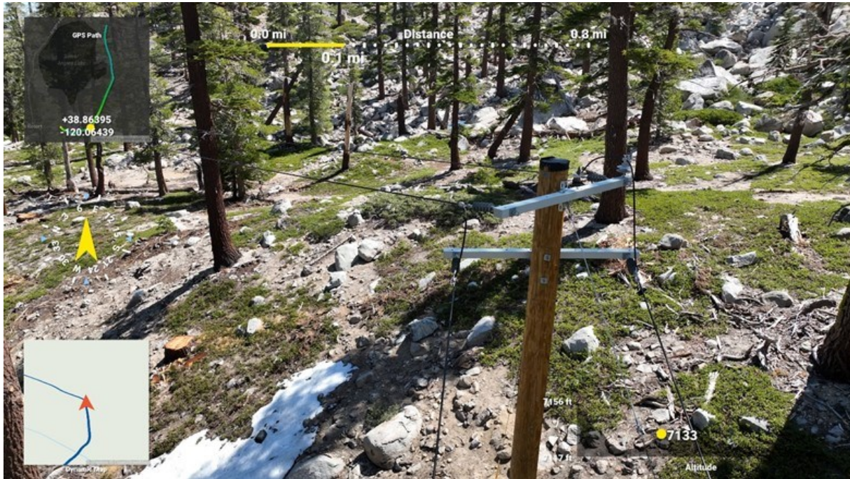
Figure 4: Example of Covered Conductor Installation (Drone Capture). Circuit ID MEY3400, Structure Number 295360.
