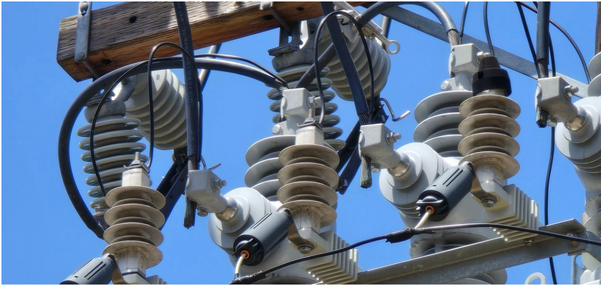
152271102-465074 – Missing Two Lightning Arrester Caps
