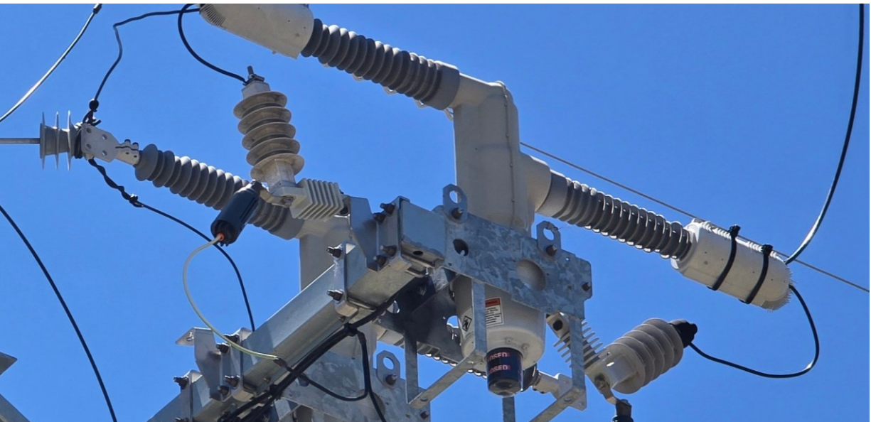
182611104-913884 – Missing 1 Lightning Arrester Cap
