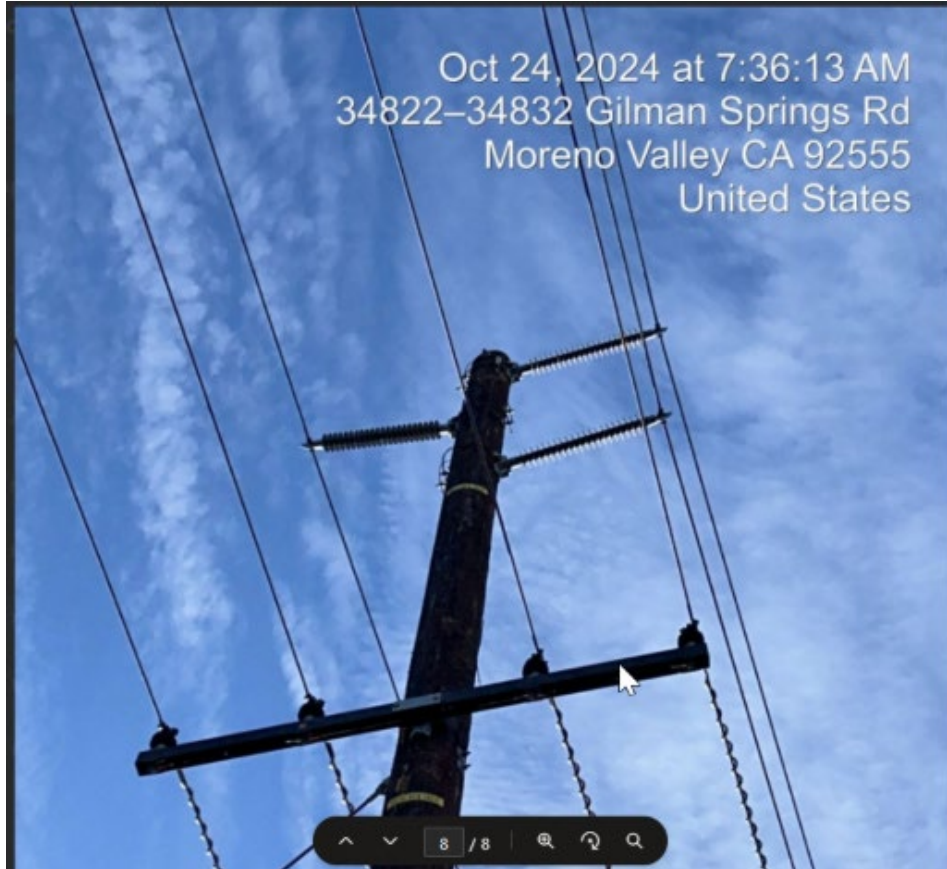
Photo 3 – Covered Conductor Installation Structure ID 4491295E
