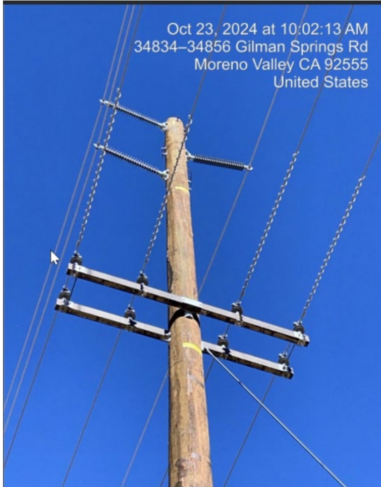
Photo 3 – Covered Conductor Installation Structure ID 4491275E
