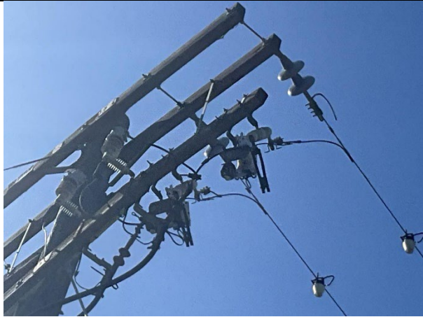
Item1IA1Img2: Dislodged lightning arrester cover
