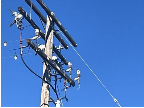
Item1IA1mg3: Dislodged lightning arrester cover
