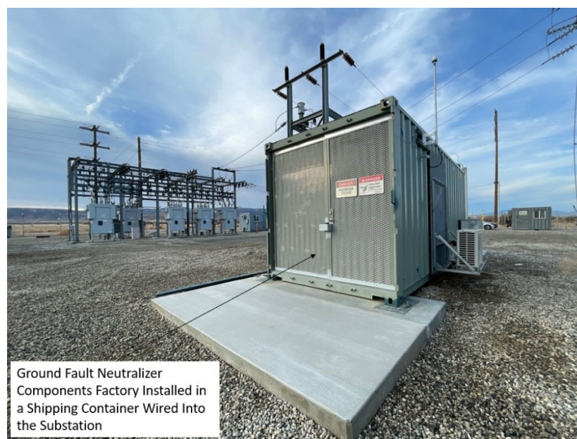
Figure SCE 8-07: Image of a Ground Fault Neutralizer
