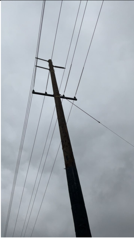
Item2IA1mg1: View showing no wildlife covers installed
