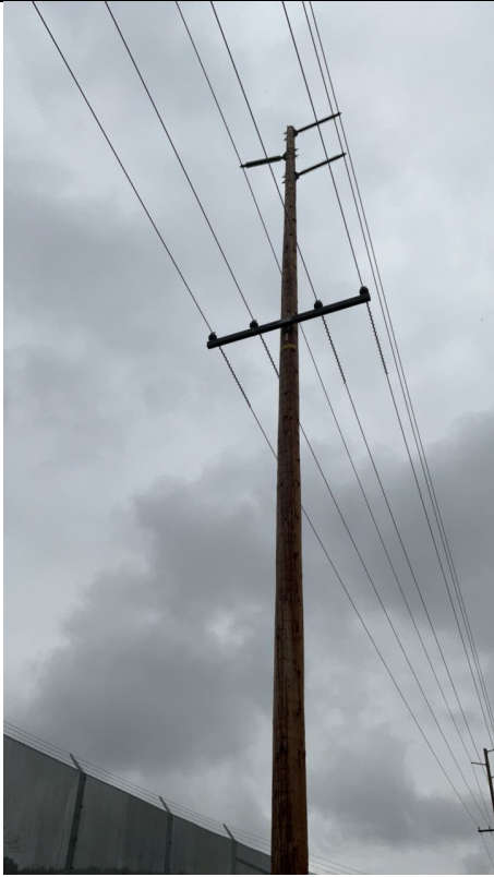
Item1IA1mg1: View showing no wildlife covers installed
