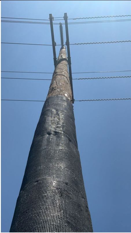
Item3IA1Img1: View showing no wildlife covers installed
