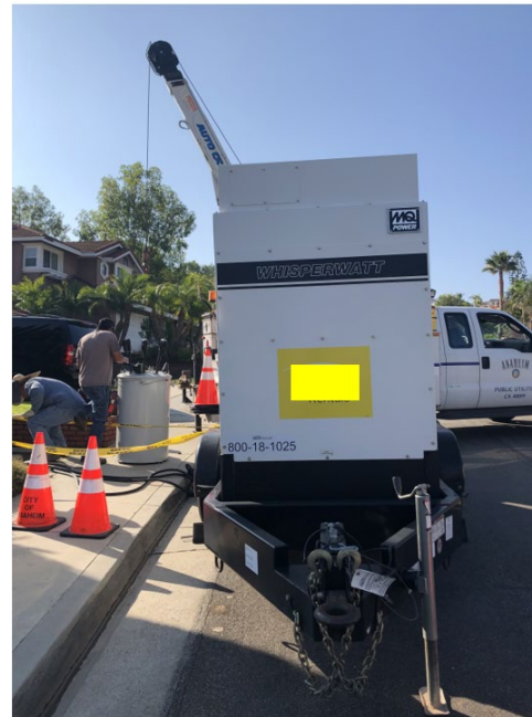
Figure 19: APU Emergency Generator
