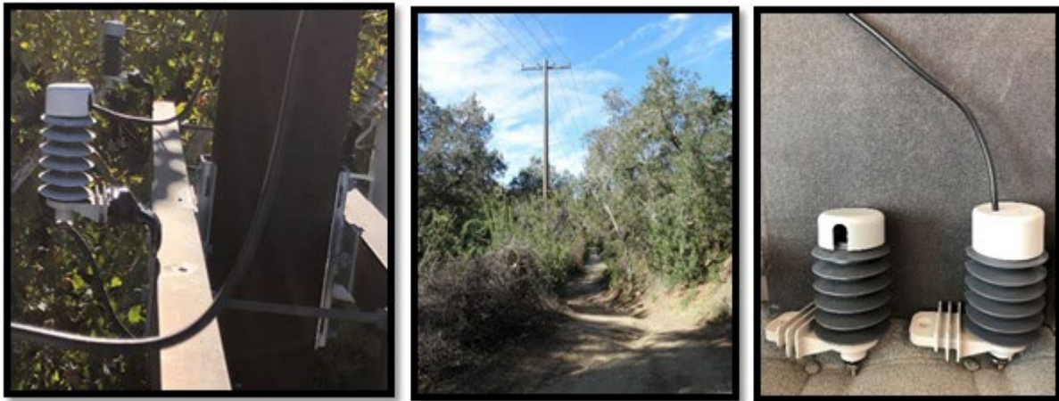
Figure 16: (a) Concealed Lightning Arrester (b) Ductile Iron Pole (c) Comparison of Lightning Arrester Models
