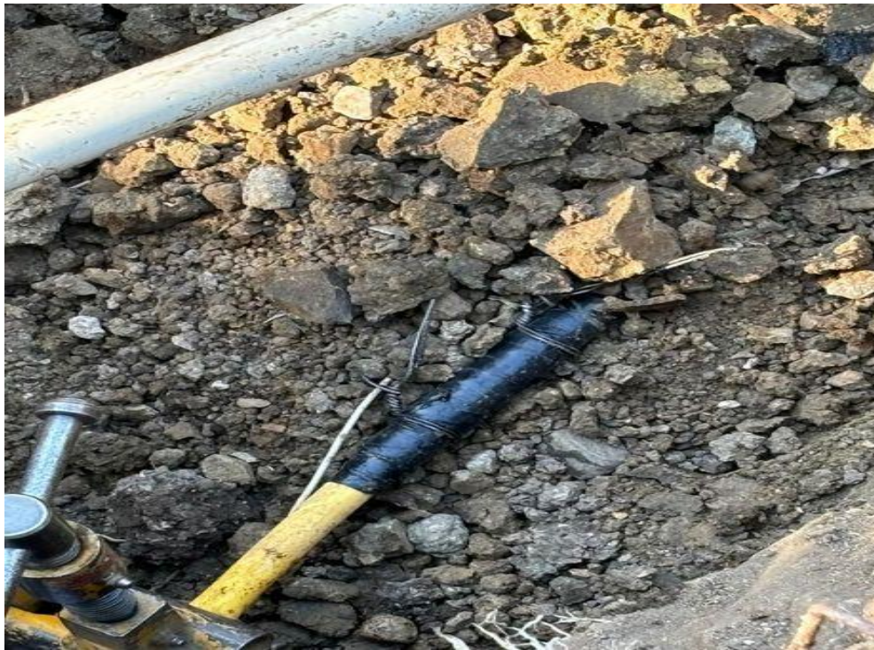
Photo 2 provided by SoCalGas as an attachment to the No-Ticket Damage Reporting Form. Photo 2 depicts the damaged gas line.
