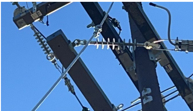
Item1IA1Img1: Down guy fiberglass strain insulator in contact with primary suspension dead-end insulator.
