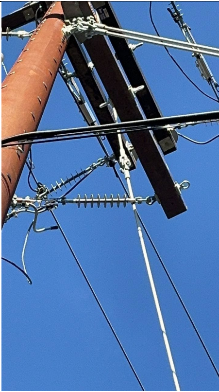
Item1GImg3: Down guy fiberglass strain insulator in contact with primary suspension dead-end insulator.
