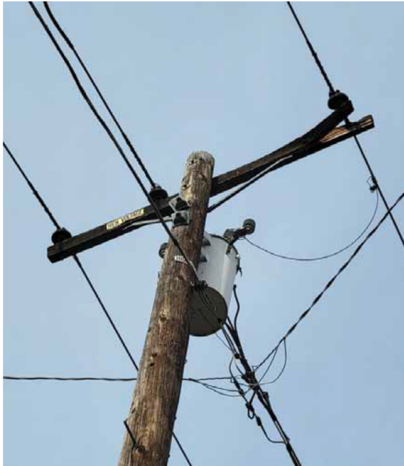
Figure 7 - Photo of damaged cross arm P516439 provided by SDG&E in their report on the December 9-11, 2024 PSPS event. The maximum recorded wind gust within 3 miles of this pole in the 72 hours prior to SDG&E's attribution of the damage time was 54.7 mph.
