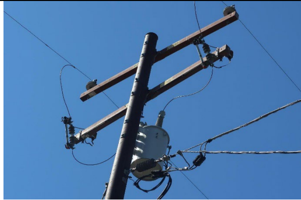
Item1IA2mg2: No avian protection on cutouts and lightning arresters
