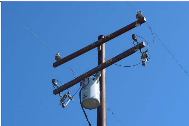
Item1IA1mg1: CAL FIRE-approved lightning arrester not installed
