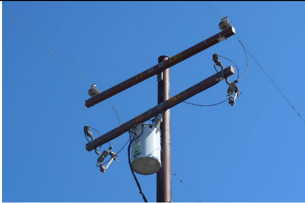
Item1IA2mg1: No avian protection on cutouts and lightning arresters
