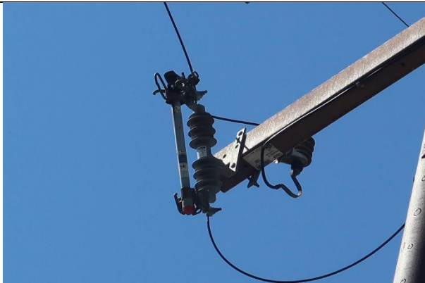
Item1IA2mg3: No avian protection on cutouts and lightning arresters
