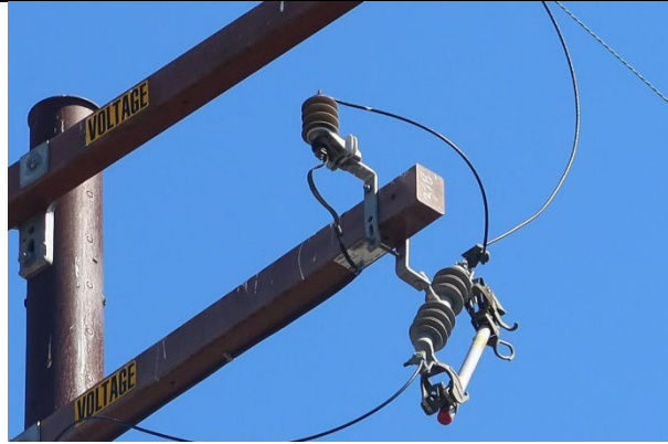
Item1IA1mg4: CAL FIRE-approved lightning arrester not installed
