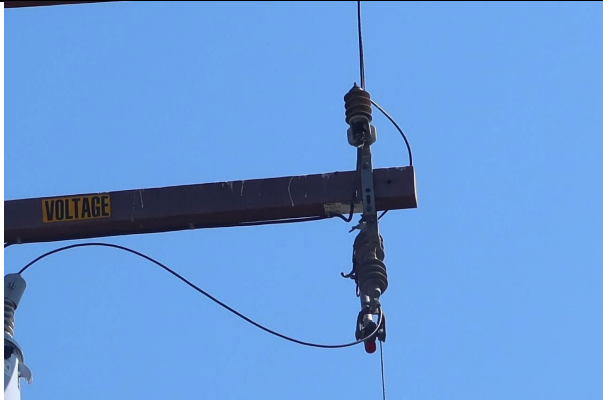
Item1IA1mg3: CAL FIRE-approved lightning arrester not installed
