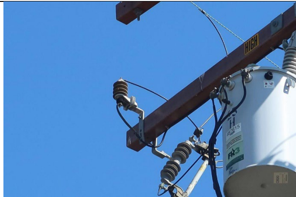
Item1IA2mg4: No avian protection on cutouts and lightning arresters
