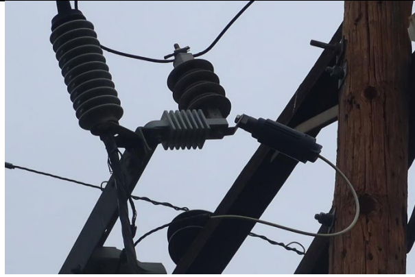
Item1IA1Img4: Missing lightning arrester cover
