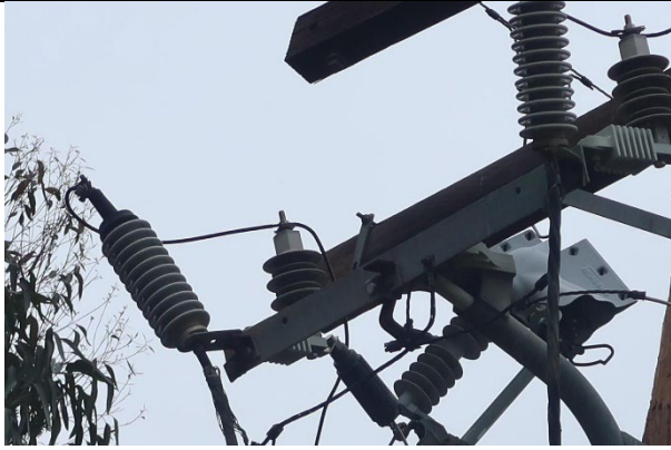
Item1IA1Img3: Missing lightning arrester cover
