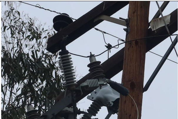
Item1IA1Img2: Missing lightning arrester cover
