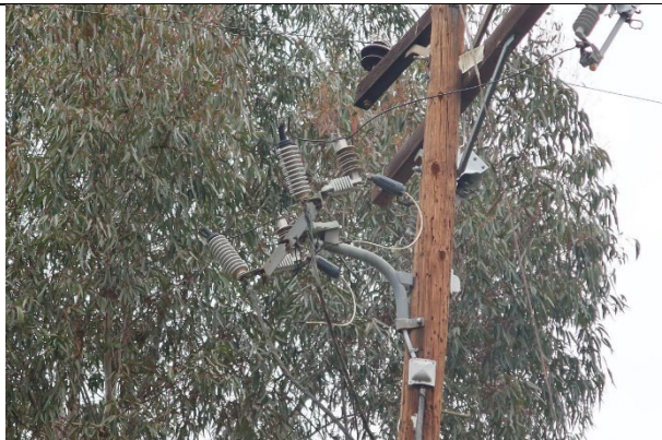
Item1IA1Img1: Missing lightning arrester cover
