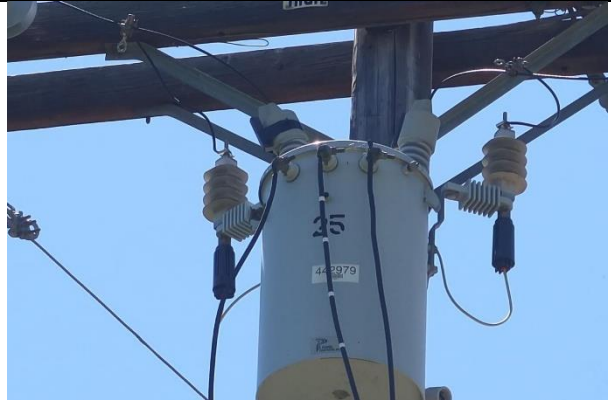
Item1IA2Img2: Lightning arresters cover missing
