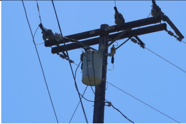
Item1IA2Img1: Lightning arresters cover missing
