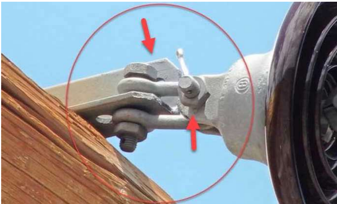
Figure 2-7: No Notification (BNC: Cotter Key Missing/Backing Out > Nut in Place > No Notification)
