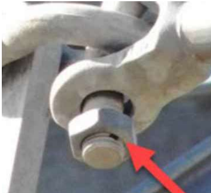
| Figure 2–6: P3 (BNC: Cottery Key Missing > Nut Backing w/ Hole Still Visable > P3)
