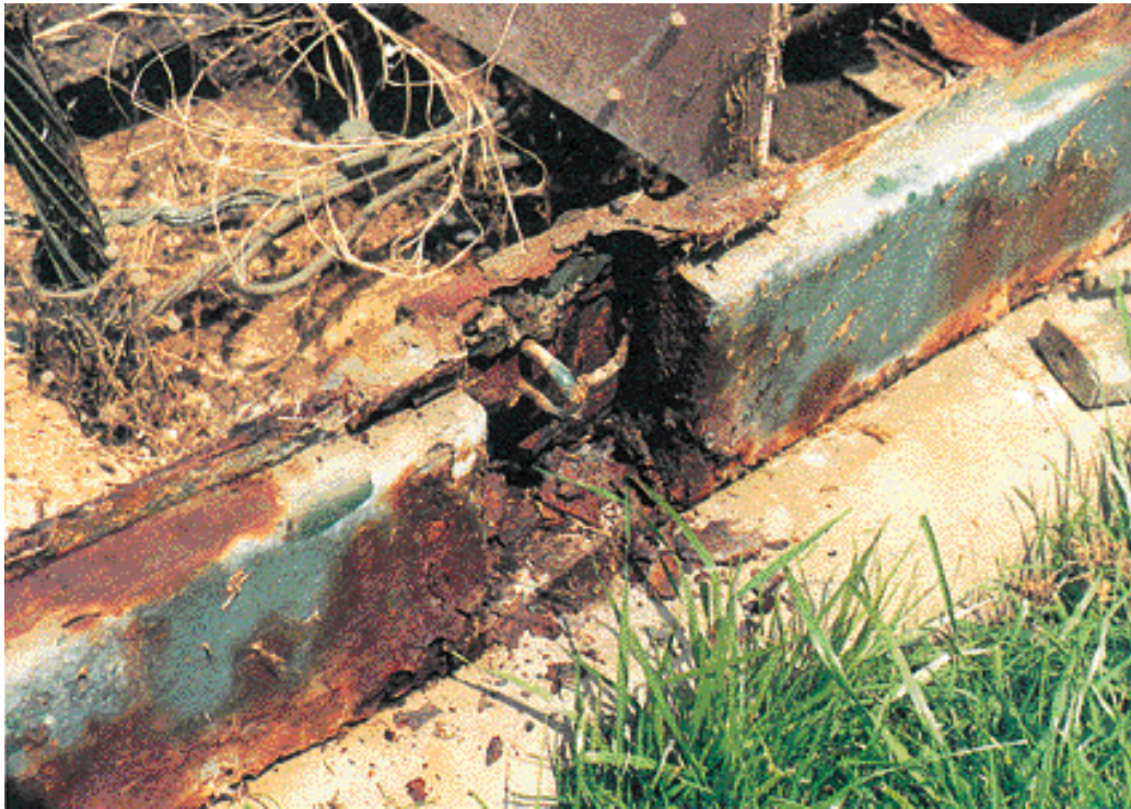
Figure 6–2: Very Heavy Corrosion of Locking Assembly
