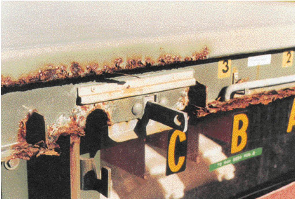
Figure 6–8: Metal Flaking Away at Nonhazardous Locations
