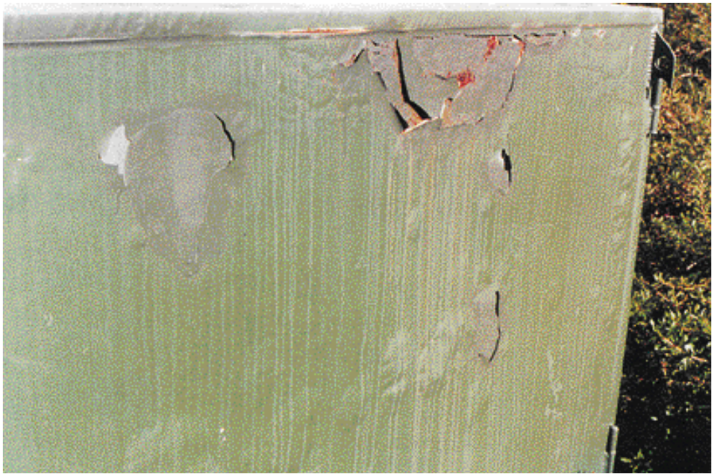
Figure 6–12: Ineffective Prior Repairs
