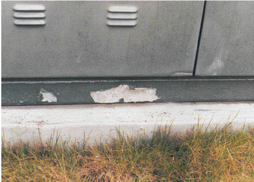
Figure 6–26: Limited Peeling of Paint
