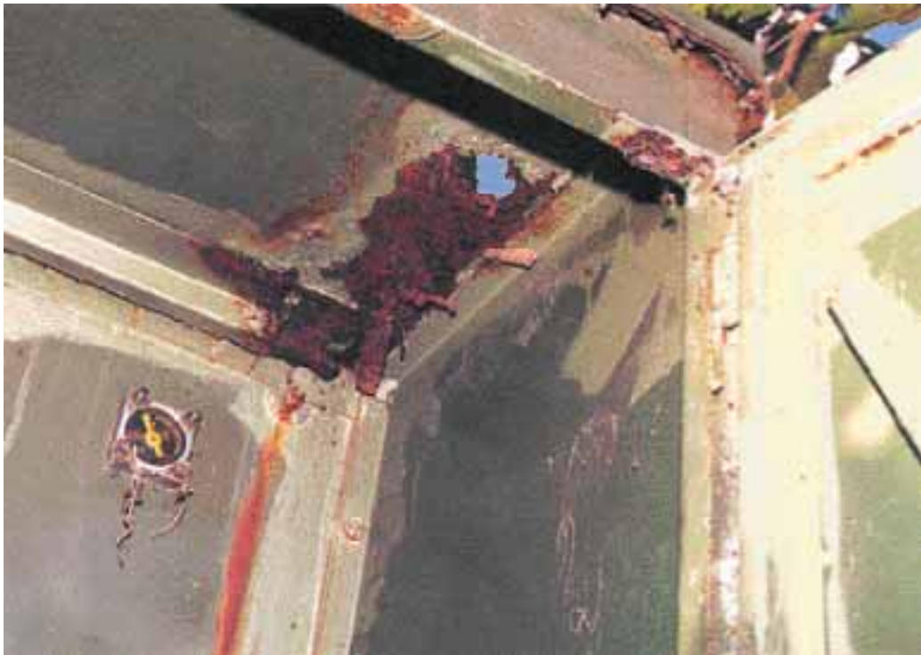
Figure 6–1: Opening Completely Through the Enclosure Wall
