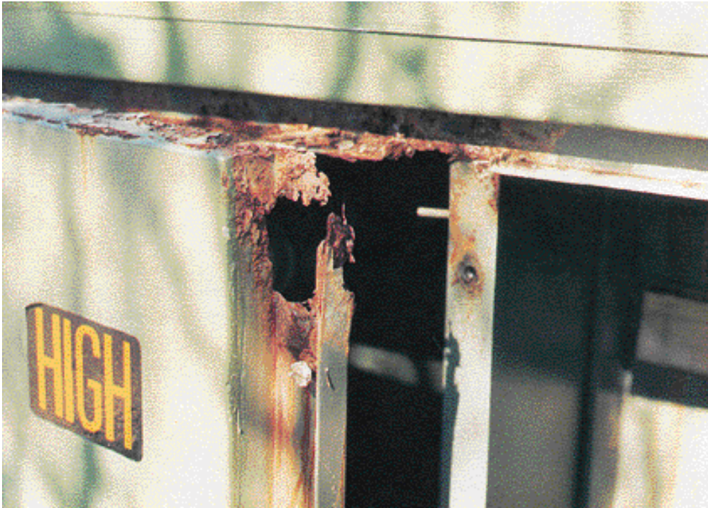
Figure 6-4: Wall Corrosion at Top of Compartment Door, Covered when Other Door Closed
