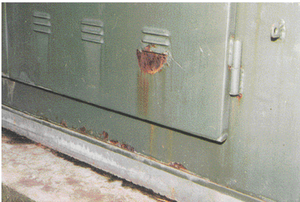
Figure 6–25: Light Corrosion at Louver Openings and at Base of Cabinet (No Serious Pitting)
