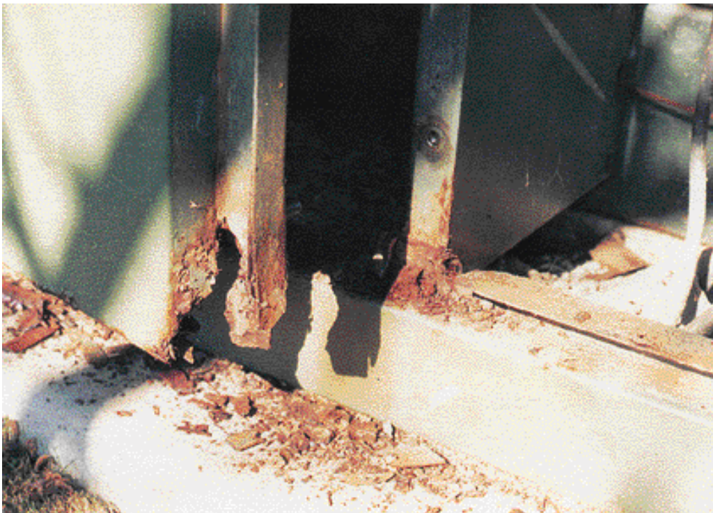
Figure 6-5: Wall Corrosion at Bottom of Compartment Door, Covered when Other Door Closed
