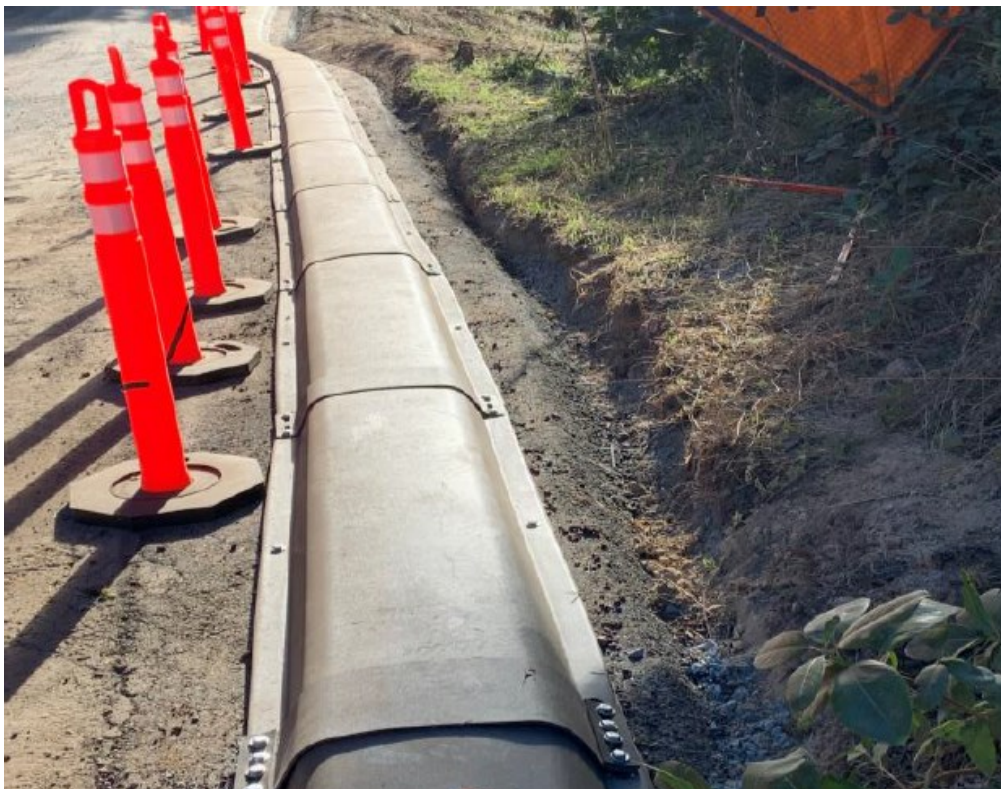
Figure SCE 8-04a: Cover Installed Over Cable Tray System from PG&E’s GLDS Pilot in Woodside
