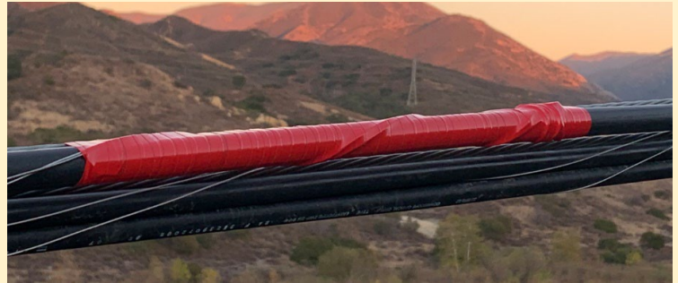
After - Snip Lashing and Tape
