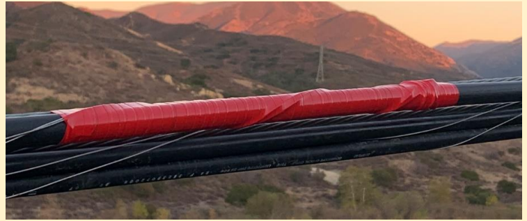
After - Snip Lashing and Tape
