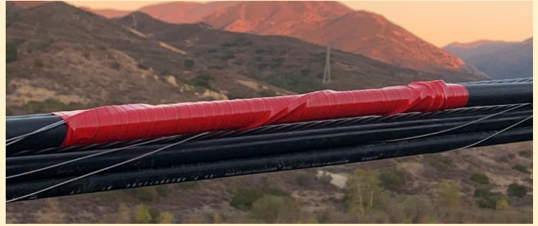
After - Snip Lashing and Tape
