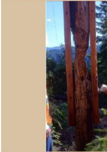
Significant reduced circumference (bear damage)
