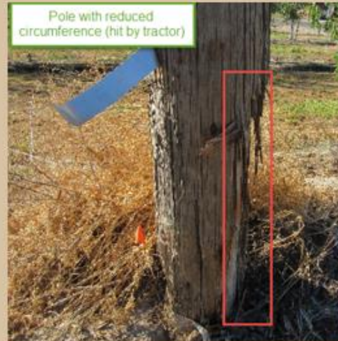
Significant reduced circumference (tractor damage)
