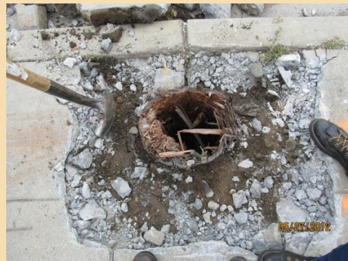
After extraction showing below ground deterioration
