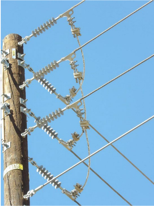
Item1IA1Img1: View of bare conductor with no covered conductor present.
