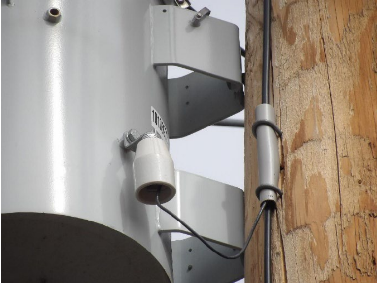
Item1IA1mg1: Loose transformer bolt hardware
