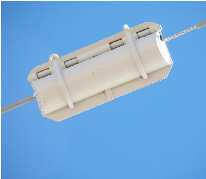
Item1IA1mg1: Close-up view of bare wire outside of wildlife cover.
