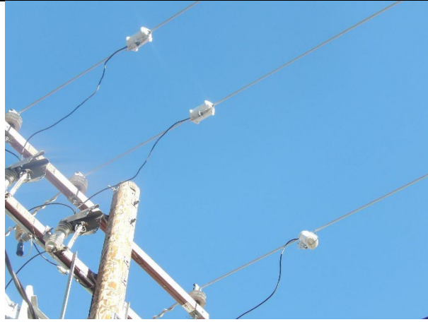
Item1IA1Img2: View of loose connector wildlife cover and adjacent connector wildlife covers.
