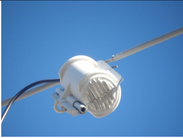
Item1IA1Img1: Close-up view of loose connector wildlife cover.
