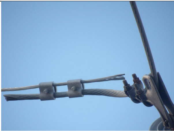
Item1IA1Img3: Close-up view of bare conductor.
