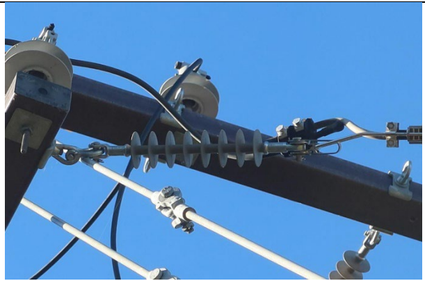
Item1IA1Img4: Down guy fiberglass strain insulator in contact with suspension primary dead-end insulator.
