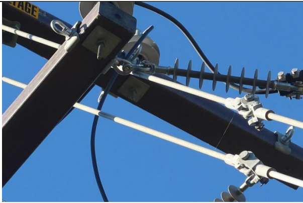
Item1IA1Img3: Down guy fiberglass strain insulator in contact with suspension primary dead-end insulator.
