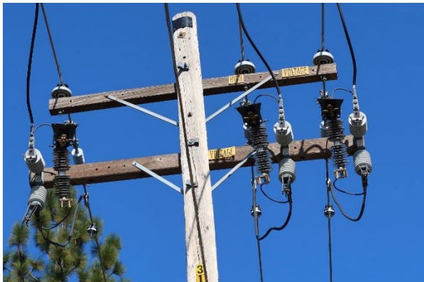
Item1IA1img1: Empty fuse cutouts
