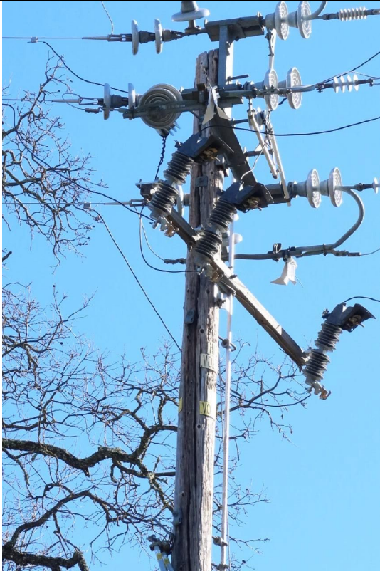
Item1IA1Img1: Empty fuse cutouts
